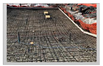
Rebar fully installed in lap pool floor, looking from shallow end down to deep end
