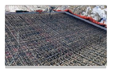
Rebar installed in lap pool floor, looking @ slope from shallow to deep end
