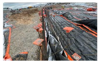
Lap pool floor covered for the weekend and wall rebar install beginning
