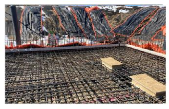
Rebar fully installed in lap pool floor
